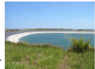
Brackish H 2 O Reservoir
