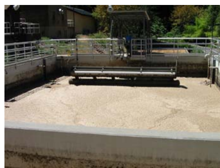
SBR basins before upgrade
