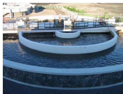
New Circular Oxidation Ditch
